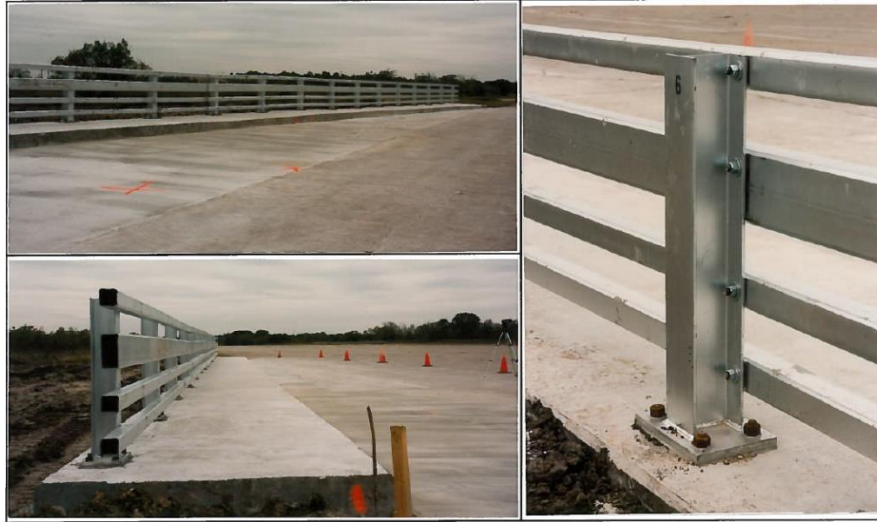
Figure 5. NETC 4-bar (SBB44b) Bridge Rail. [Kimball99]
