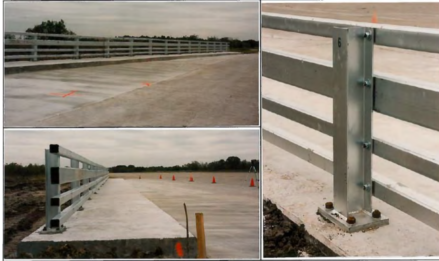
Figure 5. NETC 4-Bar (SBB44b) Bridge Rail.[Kimball99]
