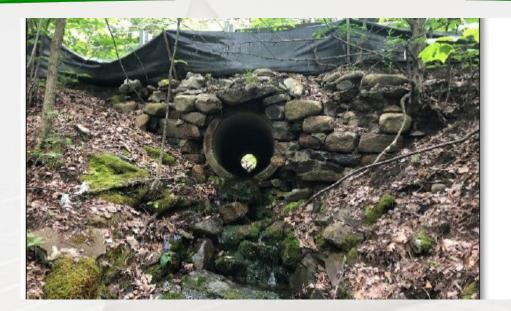
Photo 17: View of the existing 30" concrete pipe's outlet. Erosion at the crossing is problematic due to the steep topography.
