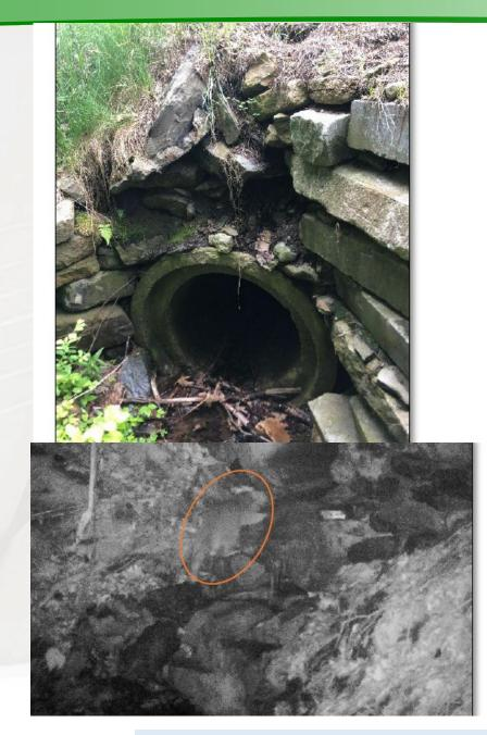
Photo 19: View of the existing 30" concrete pipe's inlet with deteriorating headwall.
