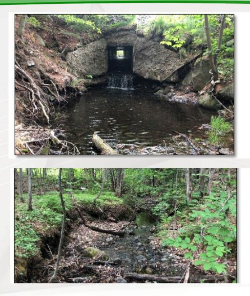
Photo 9: View of the existing 4' by 4'concrete box culvert's outlet with an approximately 18" perch, resulting in a complete barrier for aquatic organism passage. Brook trout have been observed in high densities in the scour pool. The existing structure is in poor condition with severe concrete spalling and erosion both above and below the structure's outlet.
