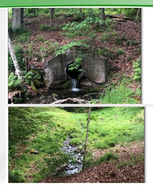
Photo 1: View of existing 36" concrete pipe's outlet with an approximately 15" perch, resulting in a complete barrier for aquatic organism passage. US Route 3 is at the top of the photo. Larger wildlife use a game trail on the right side of the photo to cross US Route 3.
