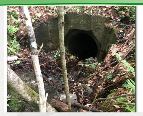
Photo 3: View of existing 36" concrete pipe's upstream inlet. Some clogging of the culvert is present because of its small size. Wildlife camera monitoring for the proposal was completed to understand existing wildlife utilization of the structure from the camera at the bottom of the photo.
