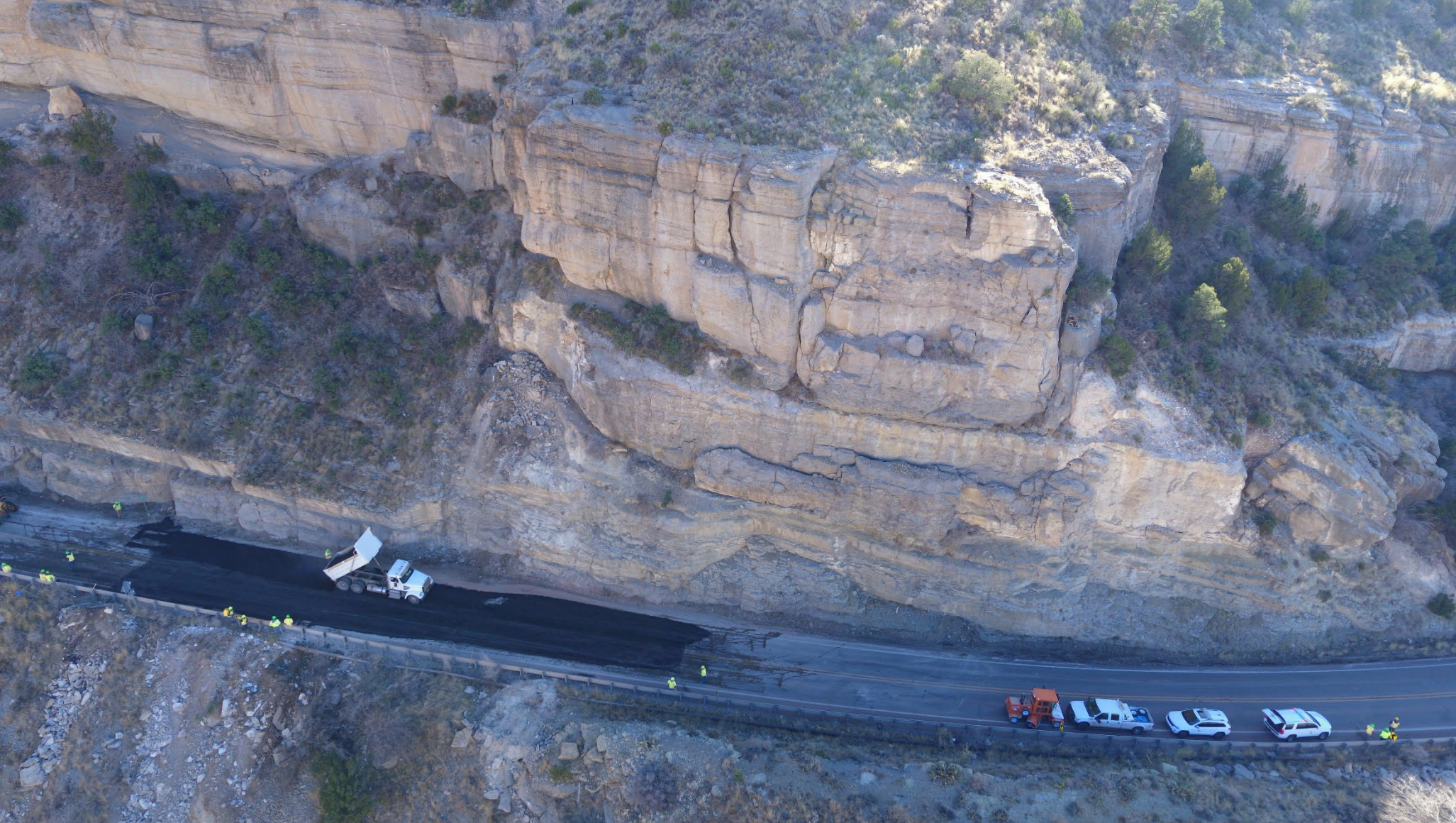
NMDOT US 82 MP 7 Rockslide Repair
