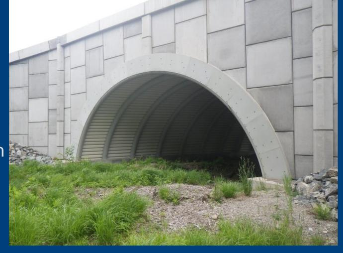
Arch bridge structure not installed specifically for wildlife passage but for fish passage
