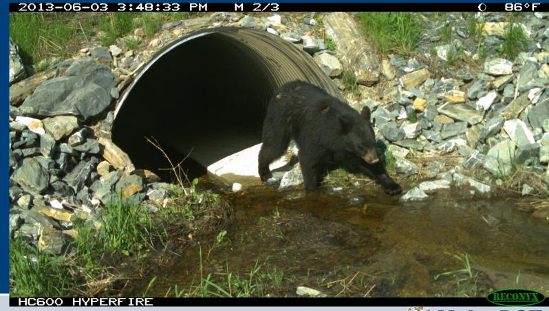
• 1.4m (54 inch) high culvert with concrete pad as shelf winter use (Cameras at each end have shown through passage)
