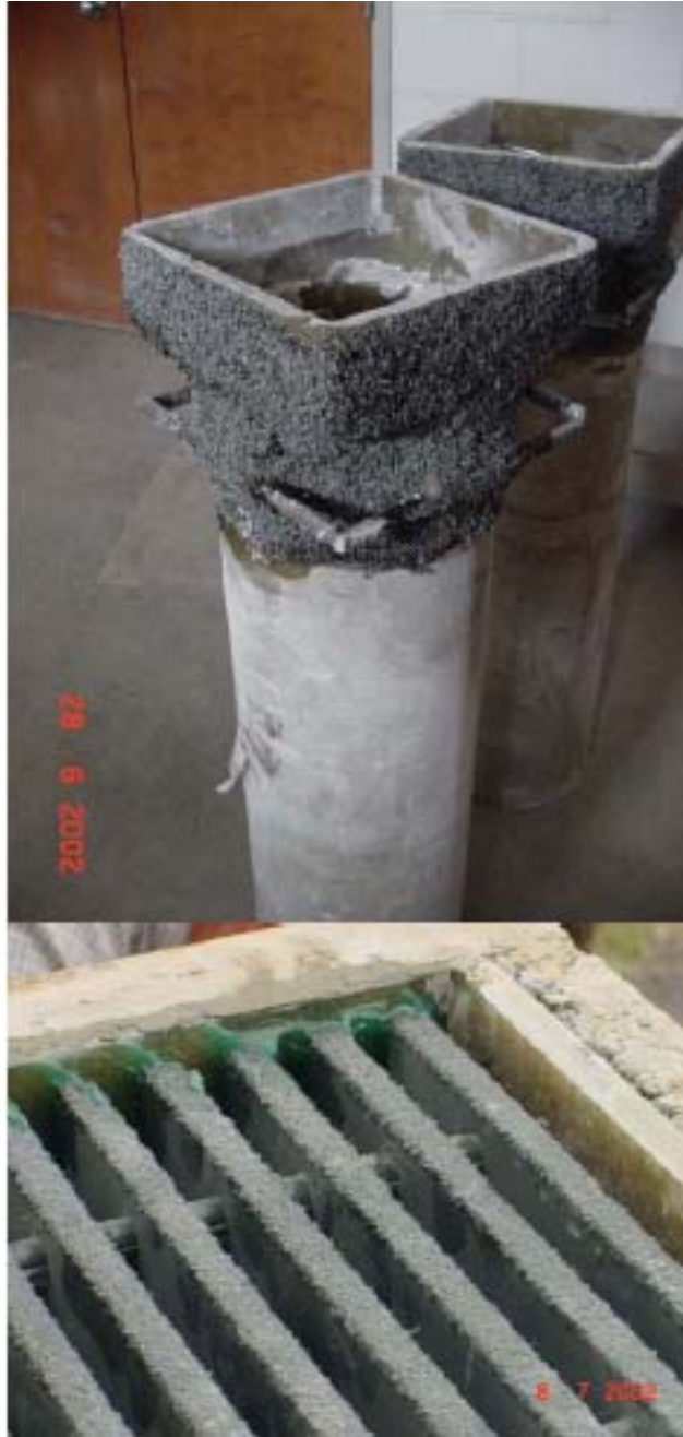
Figure 4.16 – View of finished drain prior to installation in bridge deck (Photograph courtesy of Dale Peabody, Maine DOT)
