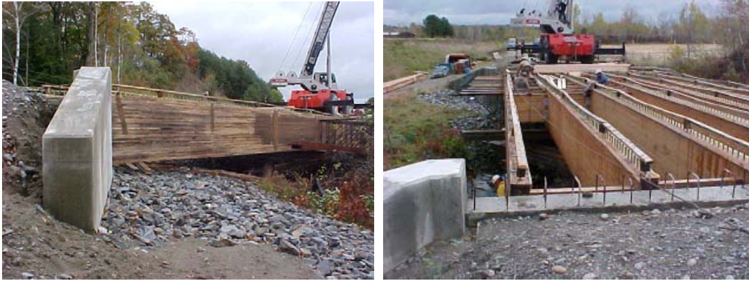
Figure 4.12 – Views of Fairfield Bridge glulams during construction (Photograph courtesy of Dale Peabody, Maine DOT)
