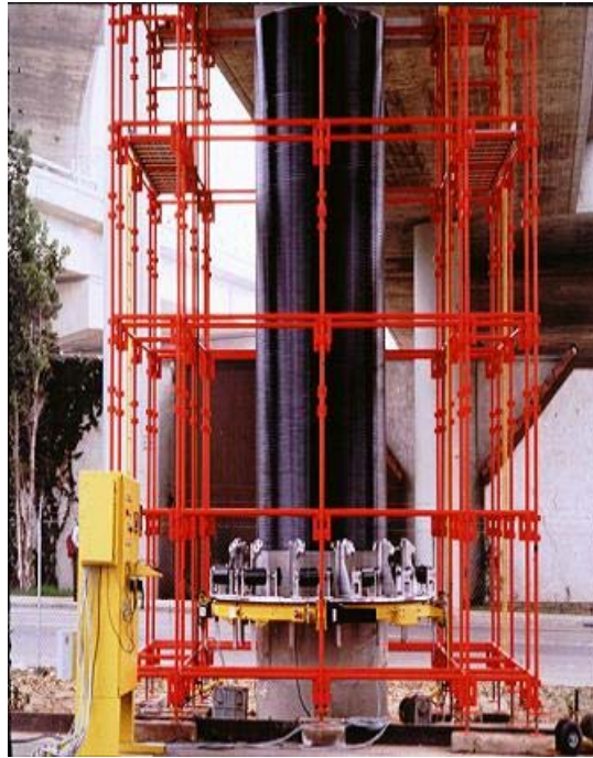
Figure 2.4 – Column rehabilitation using automated filament winding machine (source: FHWA)
