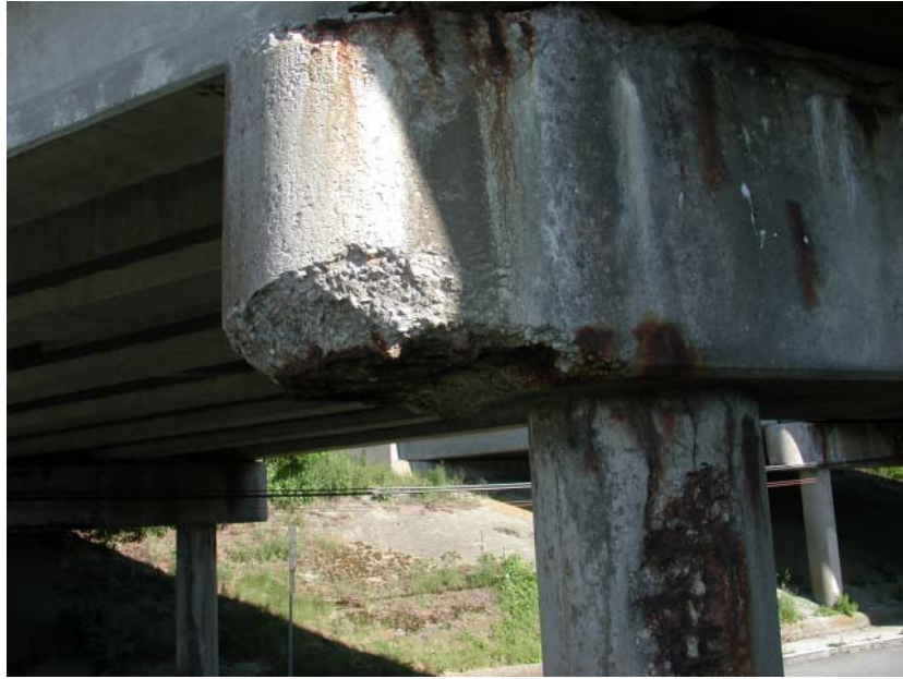
Figure 4.21 – Initial condition of pier cap (Photograph courtesy of Colin Franco, RI-DOT)
