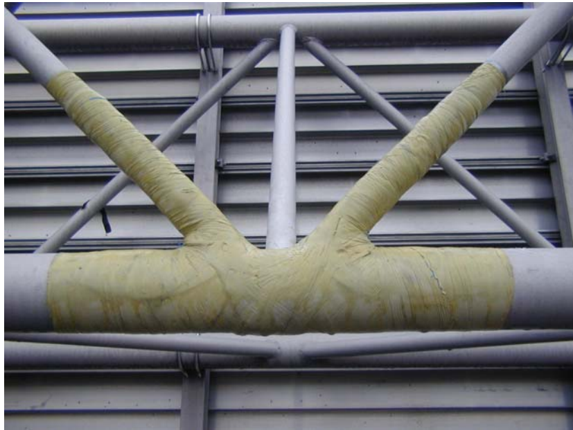
Figure 4.2 – Picture of glass FRP jacket taken toward sign (Photograph courtesy of Ned Statchen, Conn-DOT)
