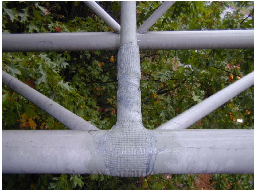
Figure 4.4 – Another view of the carbon FRP jacket in connection outside roadway (Photograph courtesy of Ned Statchen, Conn-DOT)
