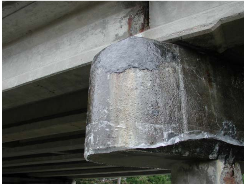
Figure 4.24 – Finished condition of encapsulated pier cap (Photograph courtesy of Colin Franco, RI-DOT)
