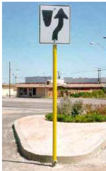
Figure 2.17 – Glass fiber-reinforced sign post (source: Highway Composites, Big Springs, TX )
