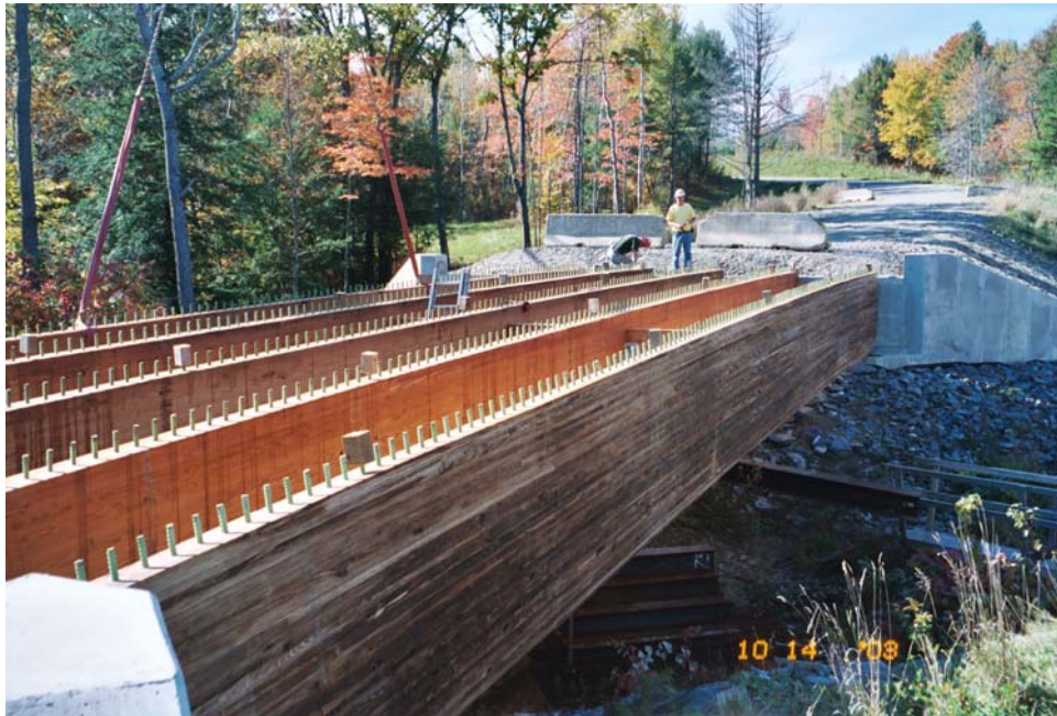
Figure 4.11 – Grouted steel dowels used to promote composite action between glulams and concrete deck in Fairfield Bridge (Photograph courtesy of Dale Peabody, Maine DOT)
