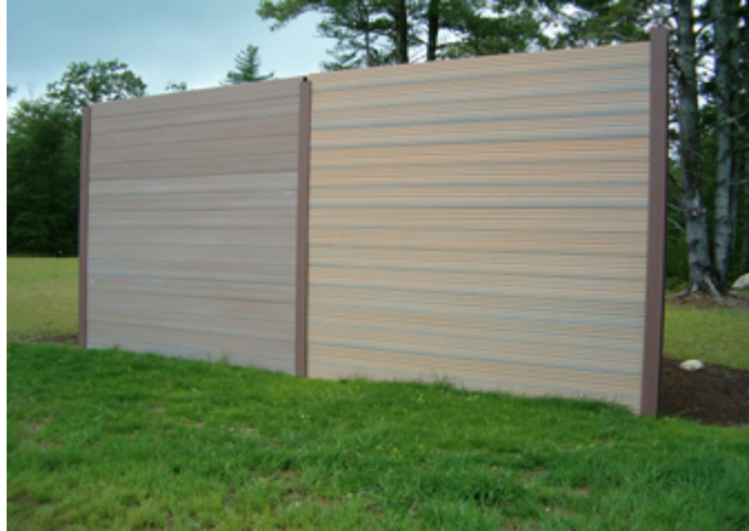
Figure 2.18 – Sound barrier fabricated from post-consumer recycled plastics – EverQuiet Wall™ (photograph courtesy of William Marcussen, New Frontier Industries, NH)
