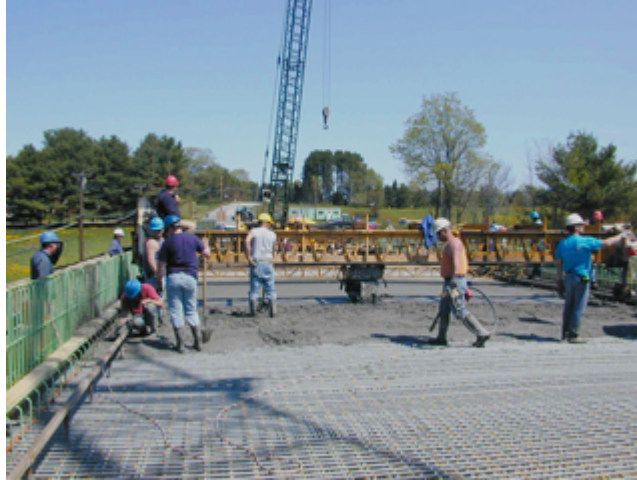
Figure 4.25 – View of deck and barrier reinforcement during deck casting (Photograph courtesy of Thomas Lackey, VAOT)
