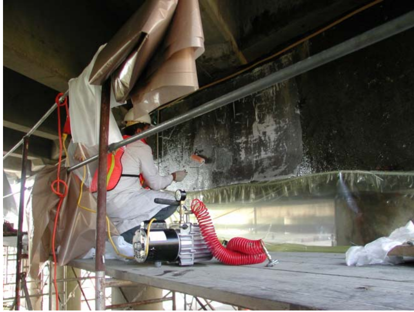
Figure 4.23 – Removal of air bubbles between bag and glass fiber fabric (Photograph courtesy of Colin Franco, RI-DOT)
