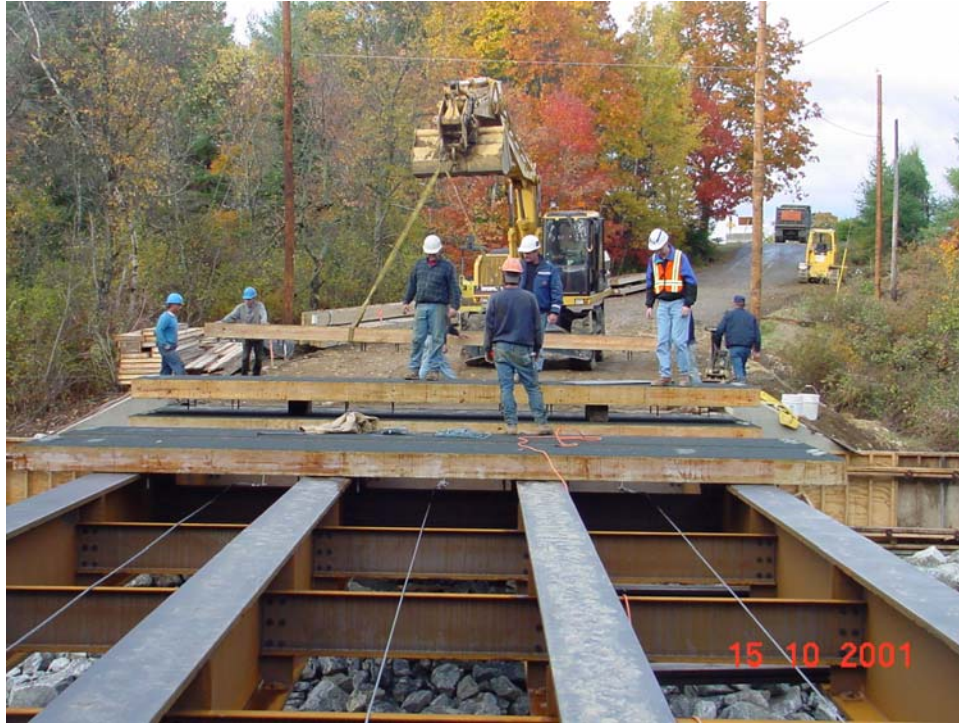
Figure 4.7 – Installation of FRP-glulam deck panels over steel girders of Skidmore Bridge (Photograph courtesy of Dale Peabody, Maine DOT)
