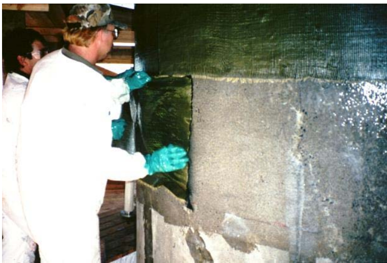
Figure 2.5 – Column rehabilitation applying FRP sheets using hand layup procedure (source: FHWA)
