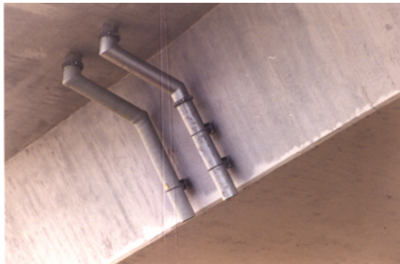
Figure 2.14 – Use of ACMs for drain and trench fabrication (trench photograph courtesy of Strongwell)
