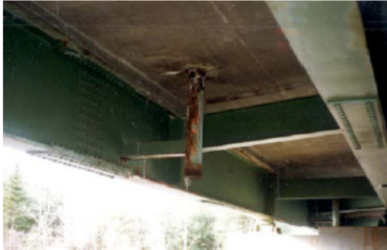
Figure 4.14 – Rusting and corrosion of steel drain under bridge (Photograph courtesy of Dale Peabody, Maine DOT)
