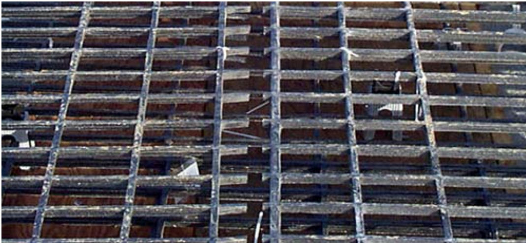
Figure 4.18 – Splice detail between adjacent NEFMAC reinforcing grids (Photograph courtesy of David Scott, NH-DOT)
