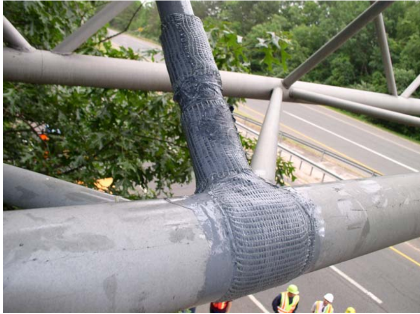
Figure 4.3 – View of carbon FRP jacket in brace connection past the right shoulder outside the roadway (Photograph courtesy of Ned Statchen, Conn-DOT)
