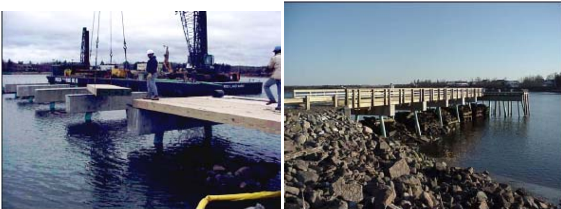
Figure 4.10 – (a) Lifting of Milbridge Pier panels during construction; (b) Finished view of Milbridge Pier (Photographs courtesy of Dale Peabody, Maine DOT)
