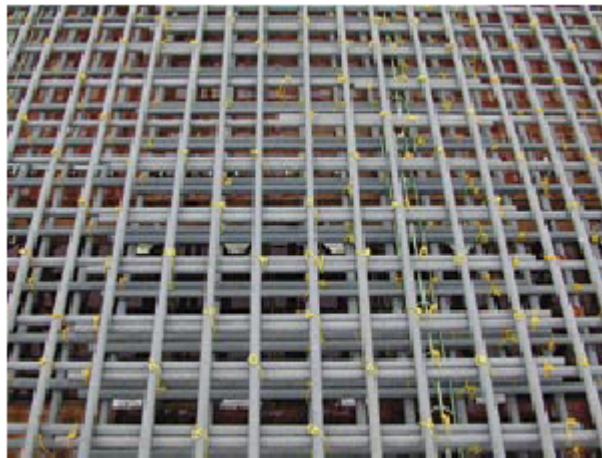
Figure 4.26 – GFRP reinforcement lap splice detail (Photograph courtesy of Thomas Lackey, VAOT)
