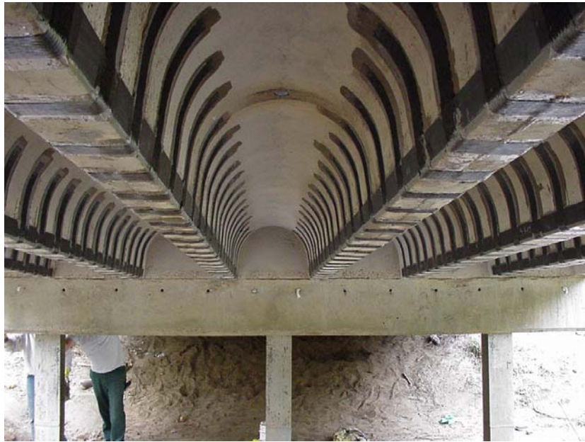
Figure 2.6 – Flexural strengthening of bridge joists using pultruded CFRP plates (Brena and Steves 2003)
