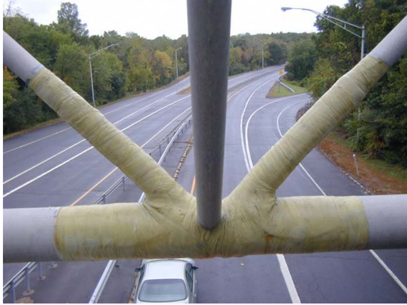
Figure 4.1 – Glass FRP jacket at bracing connection of overhead sign above left lane (Photograph courtesy of Ned Statchen, Conn-DOT)
