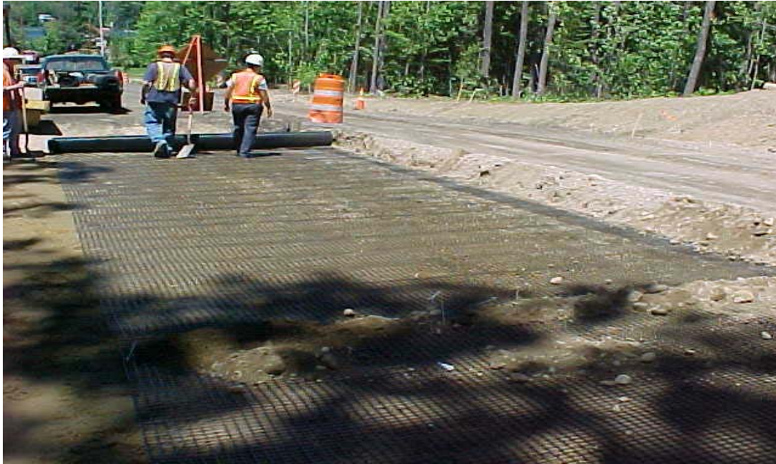
Figure 3.9 Geogrid unrolled on subgrade.
