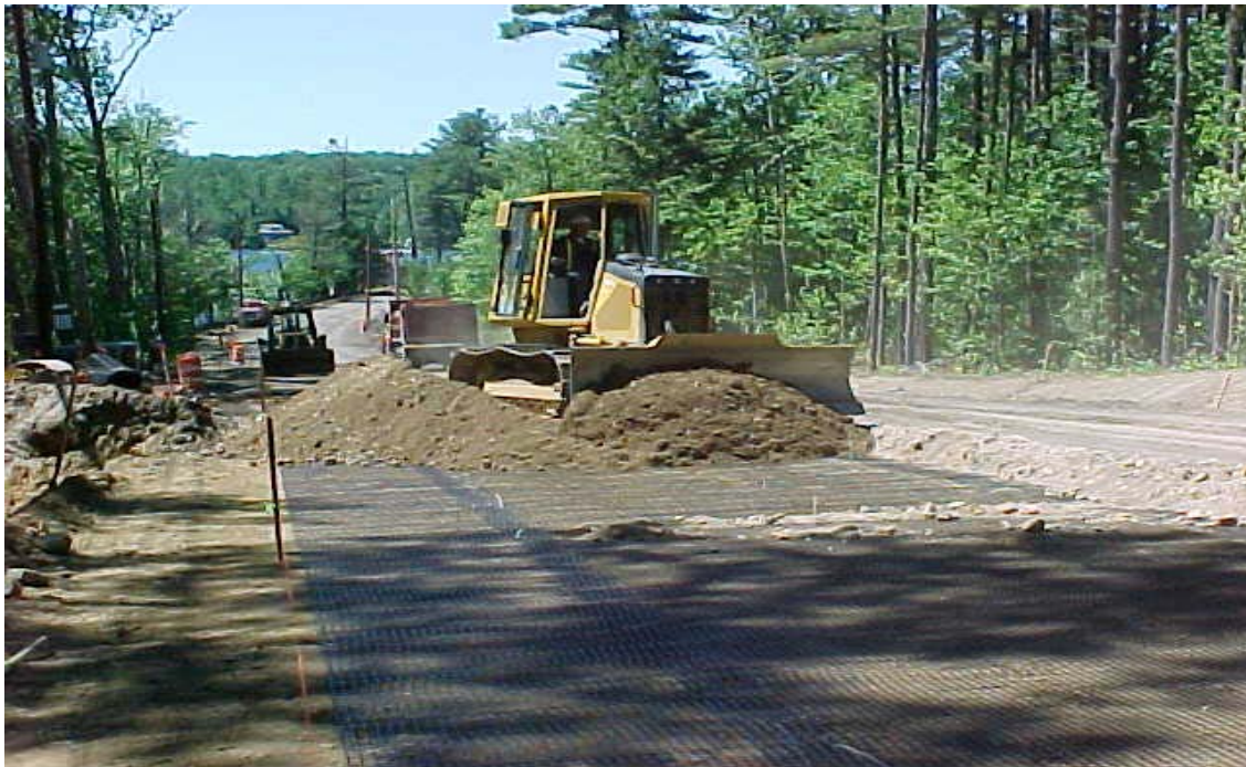
Figure 3.10 Subbase material bladed onto geogrid.
