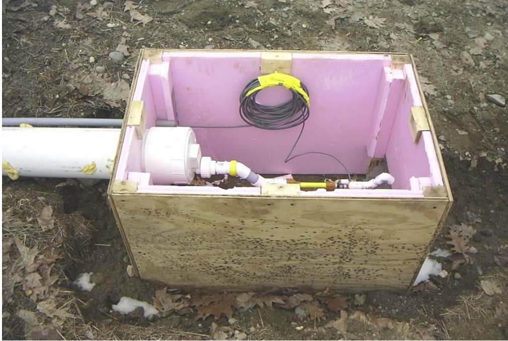
Figure 4.9 Photo of automated flow meter installation.
