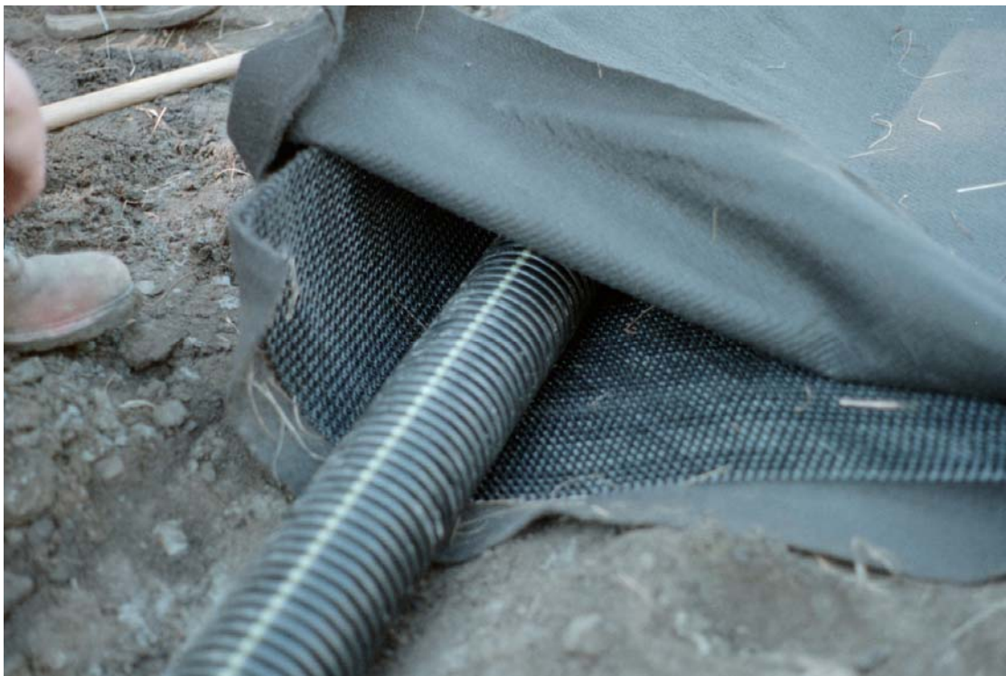
Figure 3.15 Drainage geocomposite and collector pipe.
