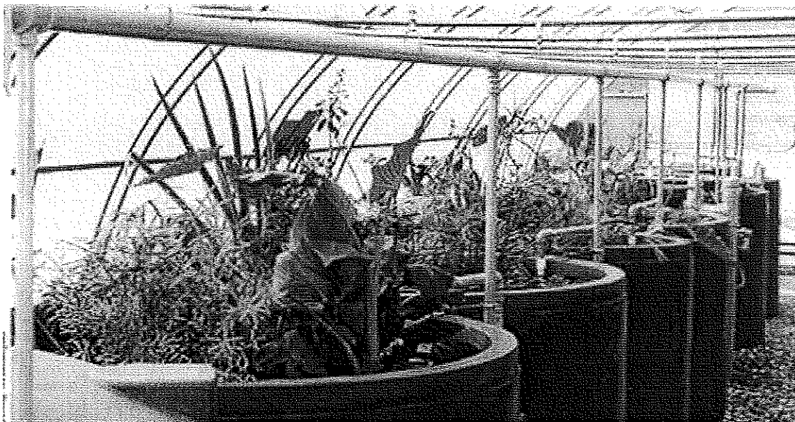
Figure 22 - Biological Wastewater System (Farrell, Van der Hoven & Olsen 2000)
