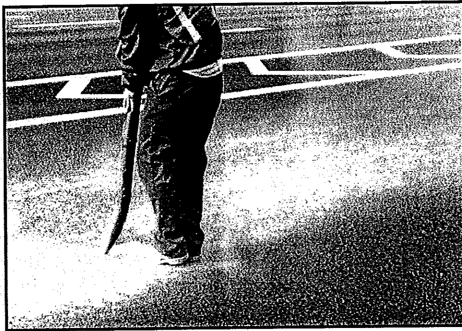
Cleaning Traffic Marking Recesses
