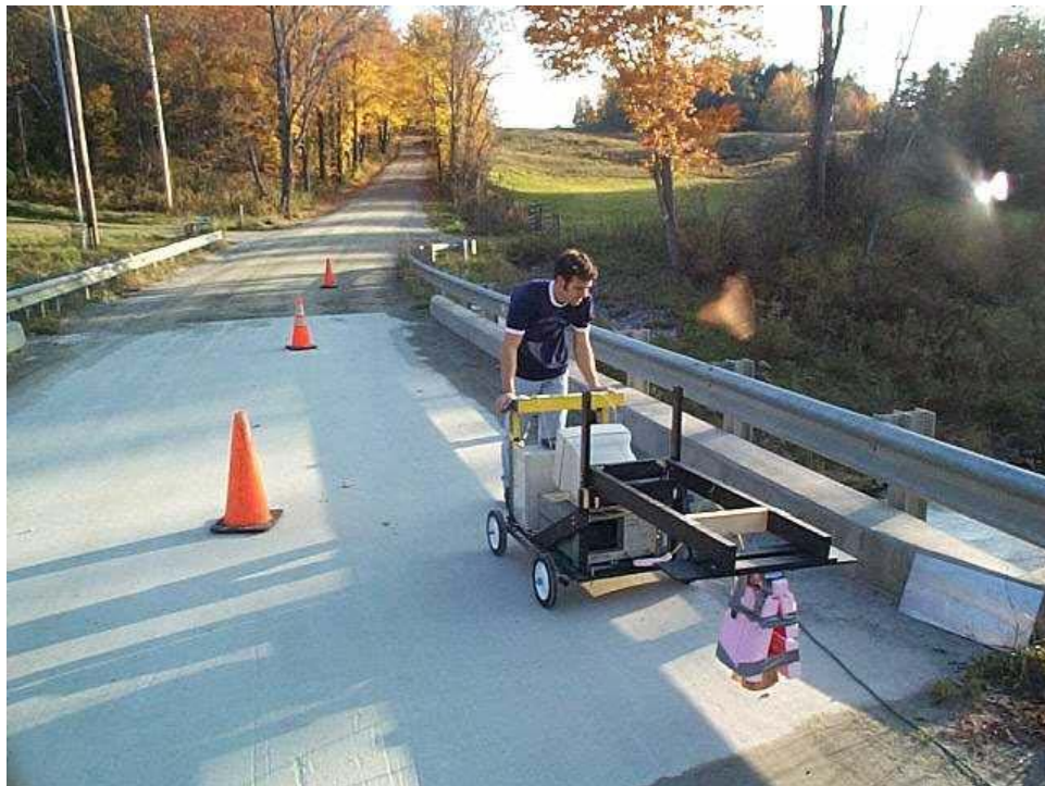
Figure 13.12 Scanning the Turkey Lane bridge deck .
