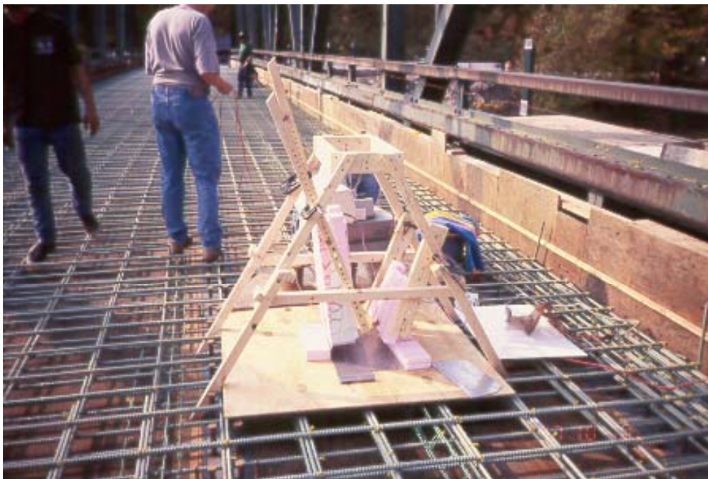
Figure 13.1 Field test conducted at the Waterbury Bridge, before a new concrete deck is placed.
