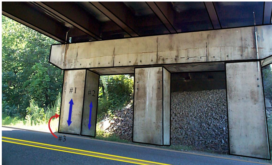
Figure 13.39. Columns of I-189 Spear St. overpass bridge in South Burlington, VT. Scan lines are indicated.
