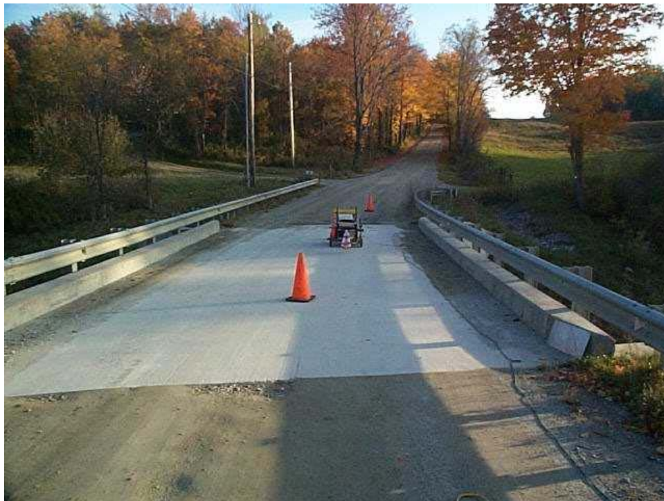
Figure 13.10. Photo of Turkey Lane bridge with GPR cart in the background.
