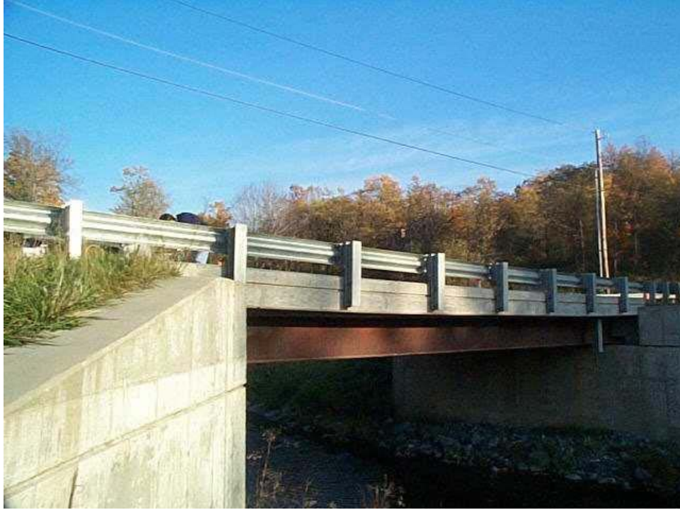
Figure 13.11 Side shot of the Turkey Lane bridge .
