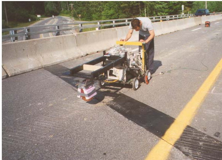
Figure 13.23 Exit 12A Bridge undergoing GPR test.
