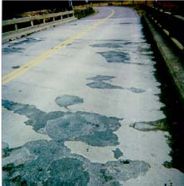
Figure 13.2 Bostwick Bridge, Shelburne, VT roadway.
