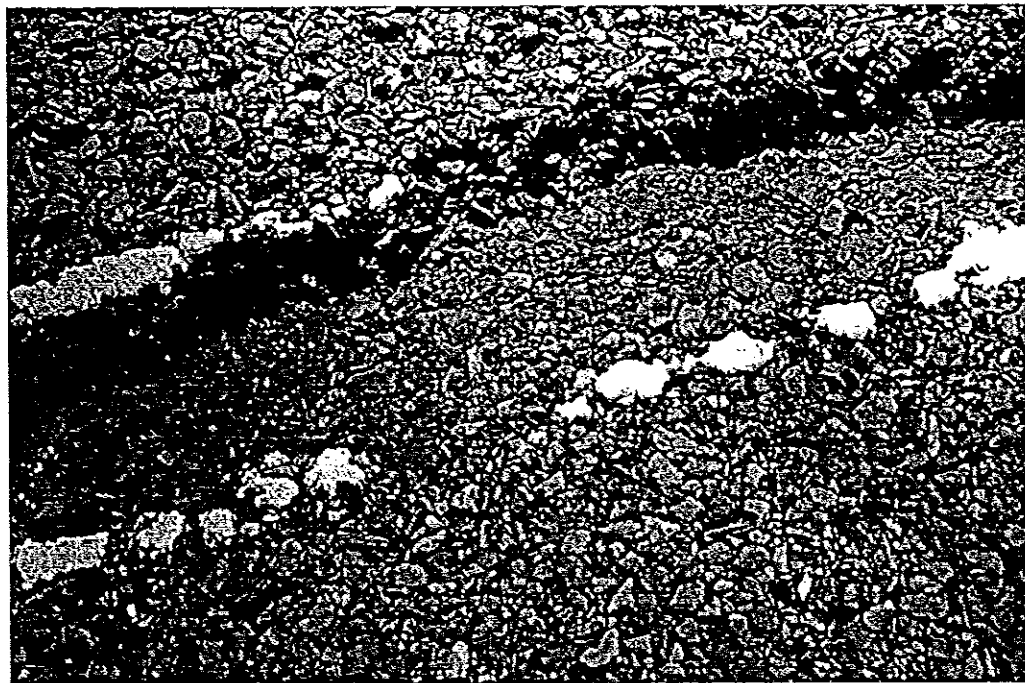
Photo D8 – I-495 NB Surface Texture and Distress @ Outer edge of Pavement (8-1000 ft)
