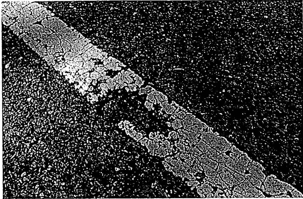
Photo D7 – I-495 NB – Distress @ Outer Edge of Pavement (6-800 ft)
