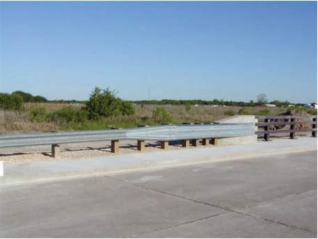
Bridge rail transitions crash-tested and qualified for use on the National Highway System; Texas Transportation Institute - $240,000
