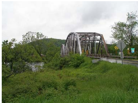
Figure 9 Candidate Bridge in Lyme, New Hampshire
