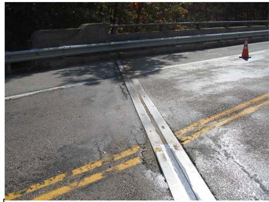
**Figure 15.** Sealant in the Rhode Island Bridge Joint
