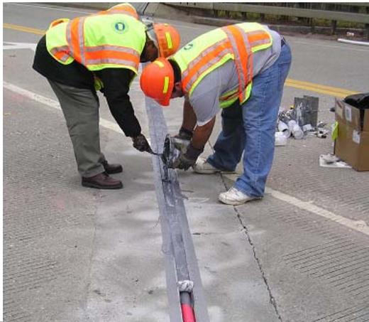
**Figure 20.** Sealing of New York Expansion Joint
