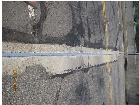
**Figure 6.** Sealant in the Connecticut Bridge Joint
