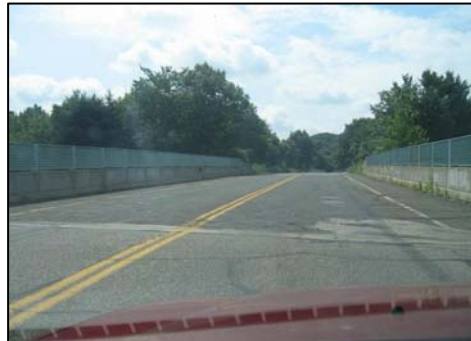
Figure 3. Candidate Bridge in Mansfield, Connecticut
