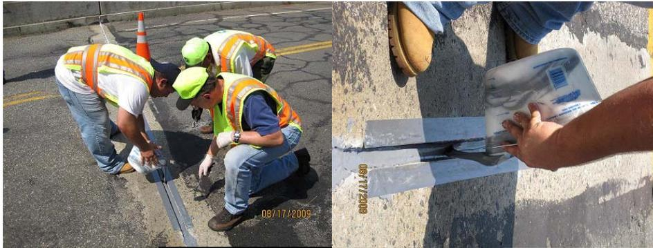
**Figure 5.** Sealing of the Bridge Joint in CT
