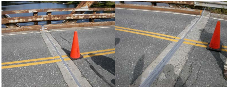
Figure 11. Sealed Expansion Joint in NH
