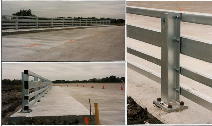
**Figure 5. NETC 4-bar (SBB44b) Bridge Rail. [Kimball99]**
