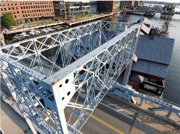
*Figure 50 - Counterweight Truss*
