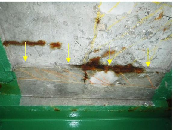
Figure 18 - Delamination along Repair due to Void / Overpour
