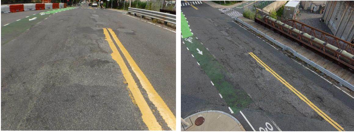
*Figure 43 - Terrestrial versus Aerial Image of Wearing Surface*
