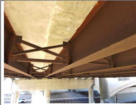
*Figure 58 - Limited View of Bottom of Girder Web and Top of Bottom Flange*
