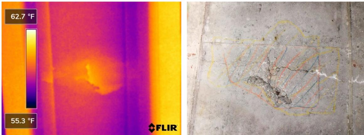
Figure 16 - Delamination with Cracking and Visible Separation
