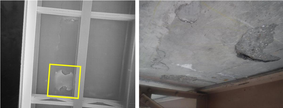
Figure 15 - Delamination without Visible Separation
