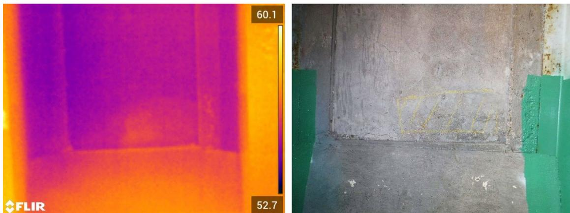
Figure 13 - Minor Delamination
