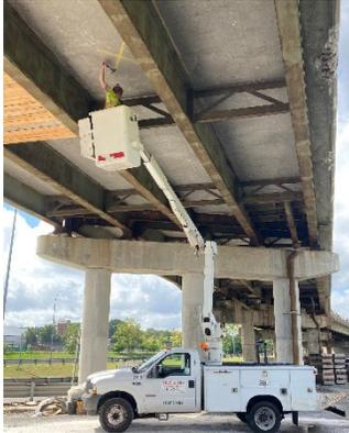
Figure 4 - Inspector Hammer Sounding Deck
