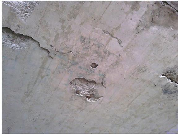
Figure 17 - Delamination with Visible Separation
