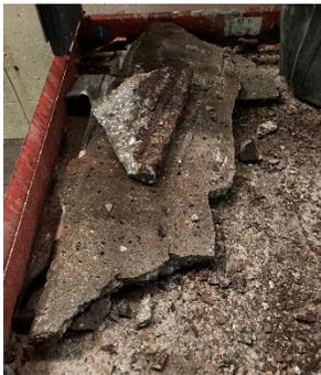
*Figure 2 - Removed Concrete from above Highway*
