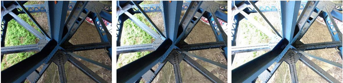
Figure 57 - Inadequate Visual Imagery due to Bridge Geometry and Lighting
