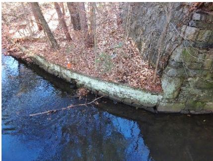
*Figure 55 - Channel Wall Deterioration Downstream of Bridge*
