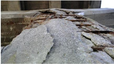
*Figure 3 - Severe Delamination / Incipient Spall*
