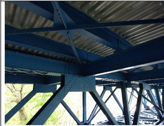
*Figure 60 - Lateral Bracing Limiting View of Stringers*
