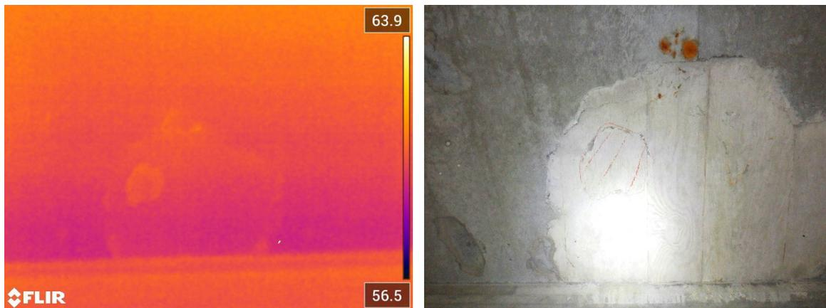
Figure 20 - Delamination within Otherwise Sound Patch
