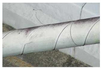
Figure 52 - Helical Bead Damage to Cable Stay
