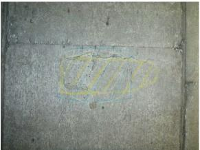
Figure 14 - Delamination with Cracking
