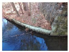
Figure 55 - Channel Wall Deterioration Downstream of Bridge
