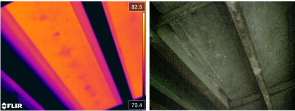
Figure 19 - Sound Patches and Delaminated Patches
