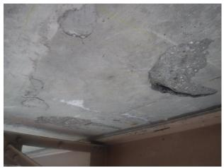
Figure 15 - Delamination without Visible Separation
