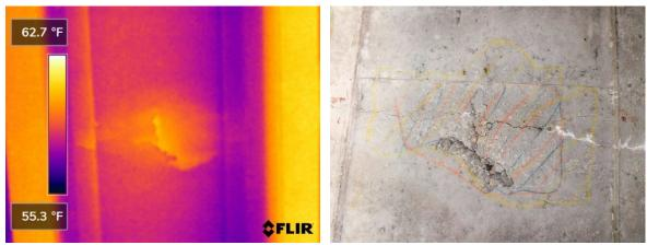
Figure 16 - Delamination with Cracking and Visible Separation
