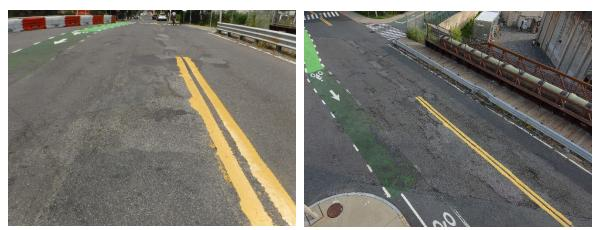
Figure 43 - Terrestrial versus Aerial Image of Wearing Surface
