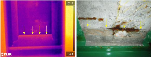
Figure 18 - Delamination along Repair due to Void / Overpour
