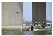
Figure 8 - UAS Operation from Boat
