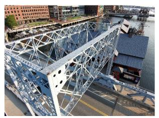
Figure 50 - Counterweight Truss
