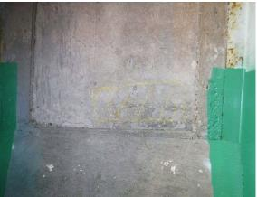
Figure 13 - Minor Delamination
