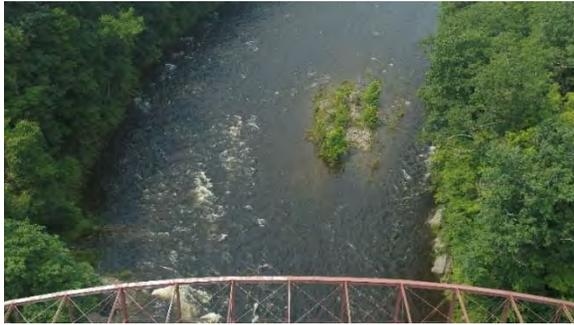
*Figure 28 - Aggradation with Vegetation Growth along Channel Upstream of Bridge*
