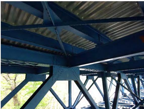
*Figure 38 - Lateral Bracing Limiting View of Stringers*
