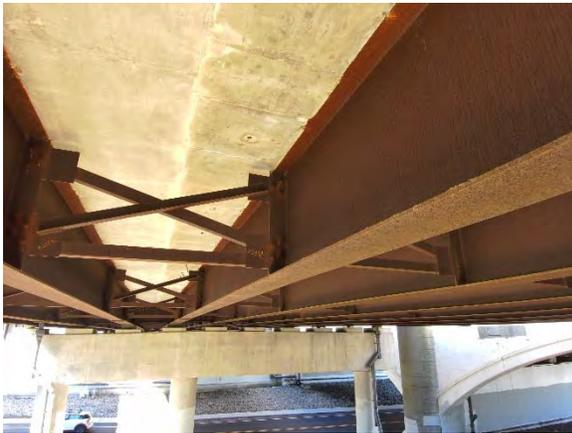
*Figure 36 – Limited View of Bottom of Girder Web and Top of Bottom Flange*
