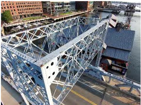
Figure 26 - Counterweight Truss
