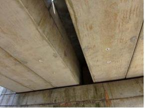
*Figure 37 – Limited View of Vertical Face at Gap between Box Beam Sections*
