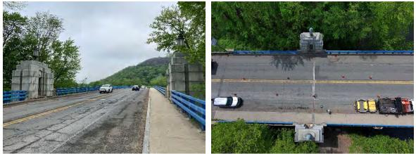
Figure 20 - Terrestrial versus Aerial Image of Wearing Surface
