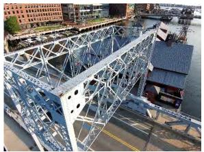
Figure 26 - Counterweight Truss
