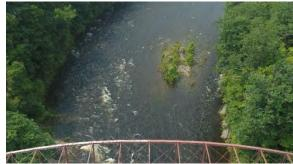
Figure 28 - Aggradation with Vegetation Growth along Channel Upstream of Bridge
