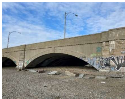
Figure 70 – East Elevation of Span 5
