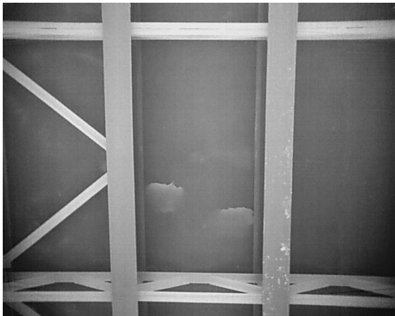
Figure 78 - Thermal Imagery captured Perpendicular to Deck near Center of Bridge Span
