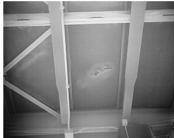
Figure 79 - Thermal Imagery Captured at Angle to avoid Pier Columns
