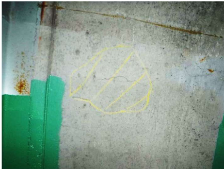
Figure 61 - Hatched Delamination
