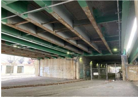
Figure 60 - Underside of Span L-M
