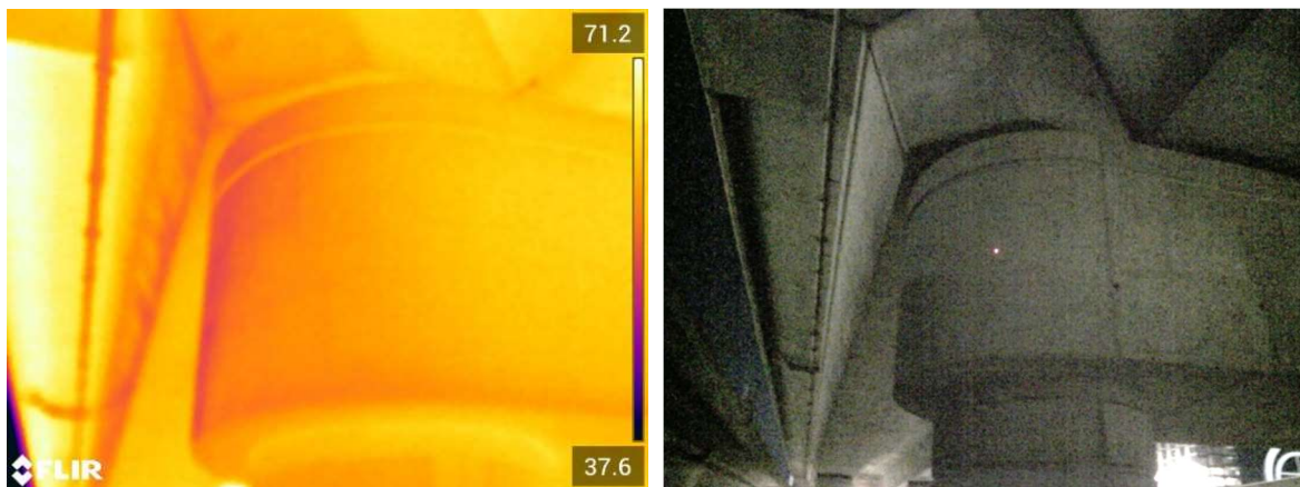
Figure 39 - Temperature Differential at Edge of Pier Cap caused by Angle of Data Capture
