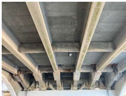
Figure 73 - Underside of Span 2
