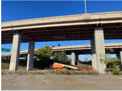
Figure 80 - Aerial Lift used for Inspection
