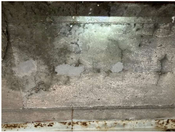
Figure 66 - False Positive from Thermal Survey
