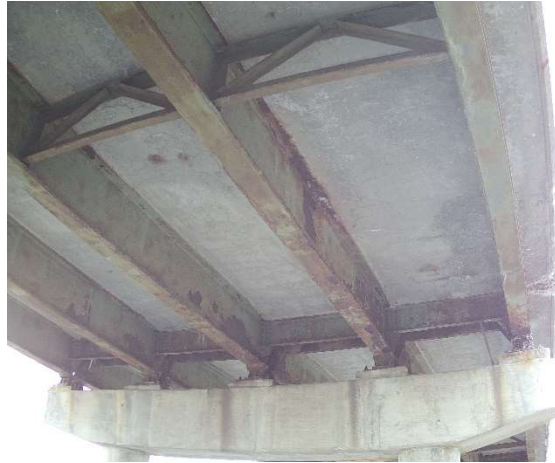
Figure 41 - Temperature Differential caused by Paint Failure along Top Flange
