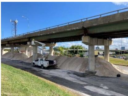
Figure 88 - BIN 4RT Traditional Inspection
