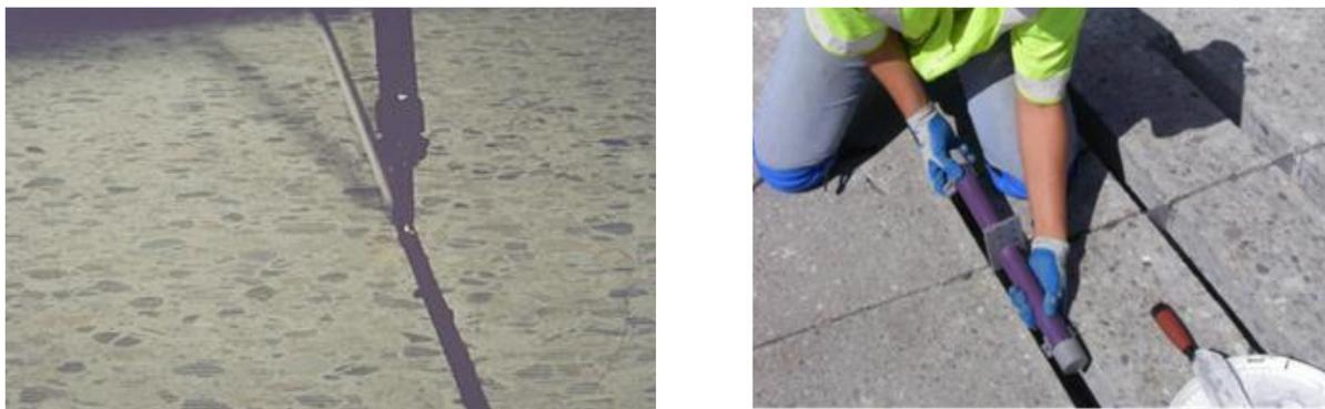
Figure 6. Joint resealing (left) and dowel bar retrofit (right) (Smith et al. 2014).
