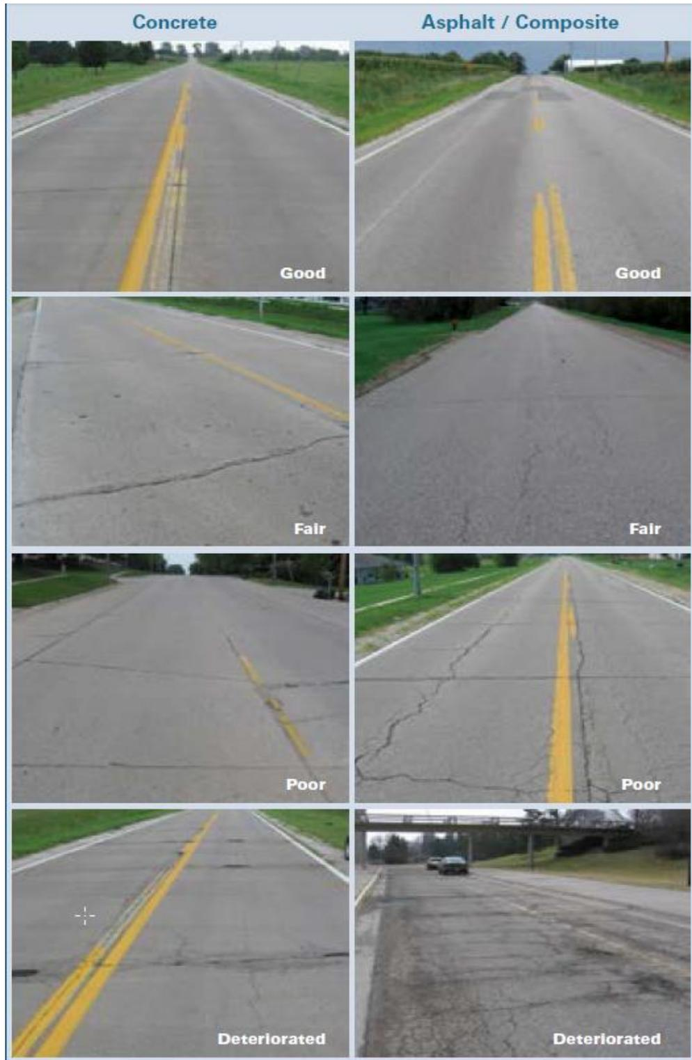
Figure 18. Example illustrations of overall pavement condition (Harrington and Fick 2014).
