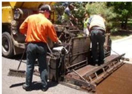
Figure 3. Crack sealing (left) and slurry seal application (right).
