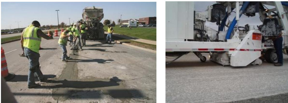
Figure 7. Partial-depth repair (left) and diamond grinding (right) (Smith et al. 2014).
