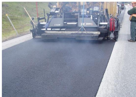
Figure 4. Chip seal application (left) (Crawford & Luce 2007) and thin HMA overlay placement (right) (courtesy of Suit-Kote Corporation).
