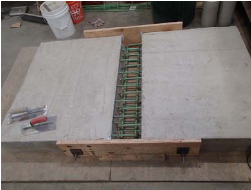
(a) Panels positioned to cast closure pour
