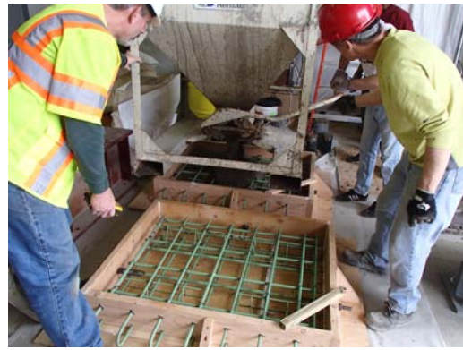
(b) Concrete placement
